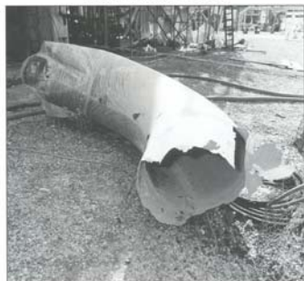
Figure 2. The 30 inch flare line elbow bent and fell to the ground, releasing the hydrocarbon
